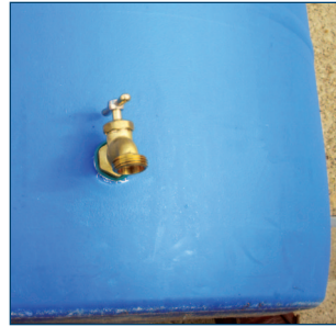
Figure 17. Hose bib facing down.
