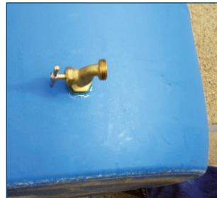
Figure 18. Hose bib facing to the side.
